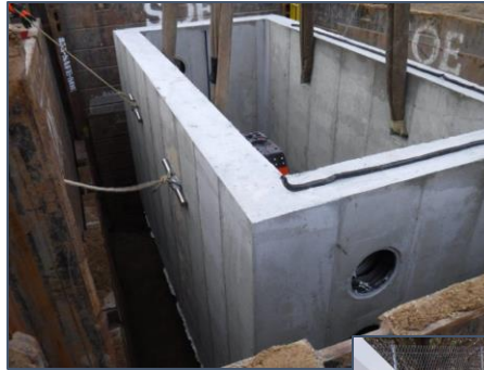
Vault Installation
